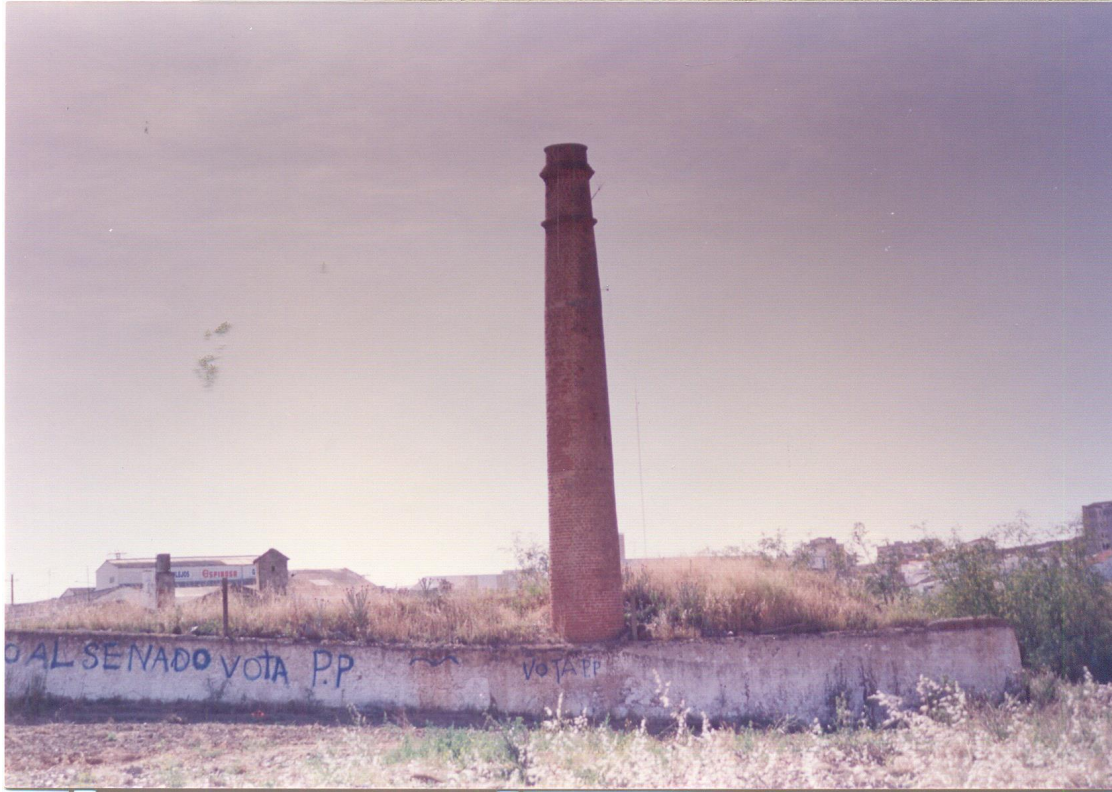
Fig. I. The chimney in the 90s. (Photo: Municipal Historical Archive of Mérida).
