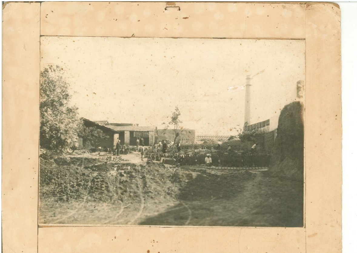
Fig. V. View of the chimney in its original context. Photograph courtesy of Juan del Río Gutiérrez.
